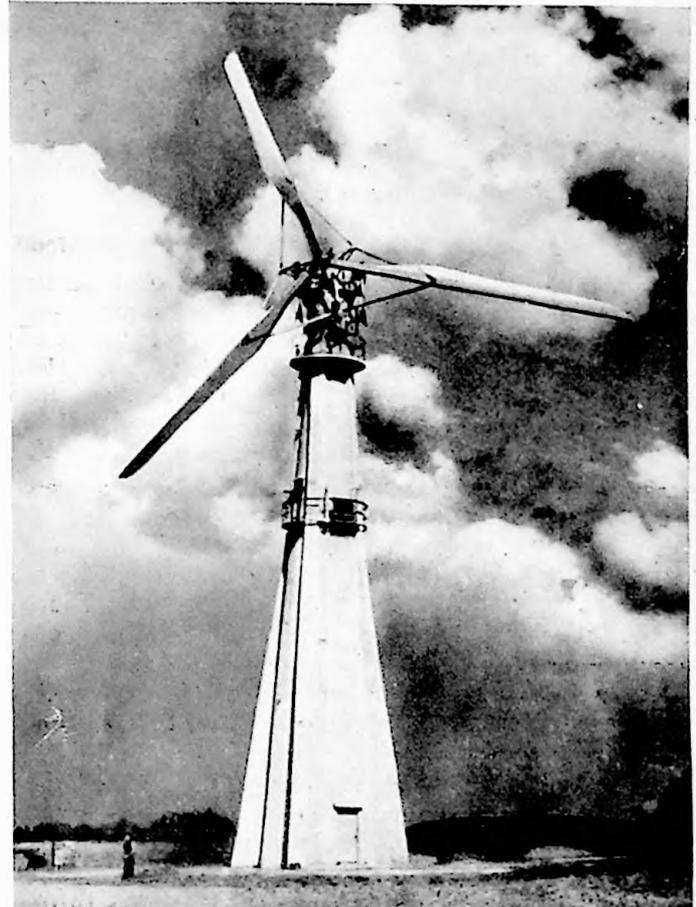
Fig. 8.—70kW wind-driven generator. (F. L. Smidth & Co. Ltd., Copenhagen.)
