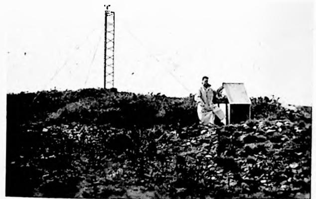
Fig. 4.—Coal-bunker housing recorder for 15-ft. lattice tower installation—St. Agnes Beacon, Cornwall.
