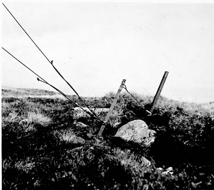
Fig. 2.—Double-picket anchorage.
