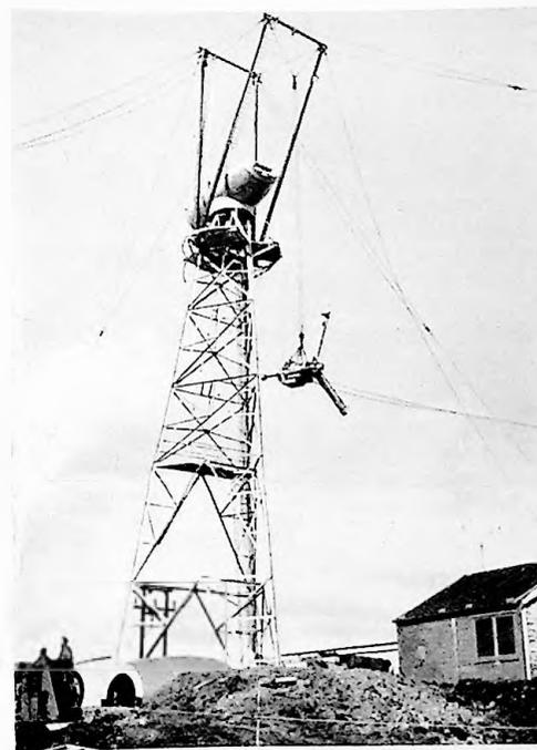
Fig. 6 A stage during construction, showing the hub and gearbox being lifted into position in the nacelle. The top half of the nacelle can be seen lying on the ground at the foot of the tower.
