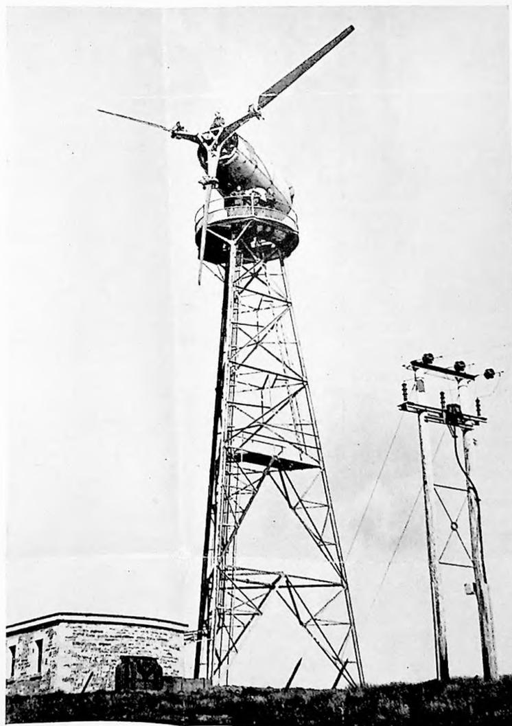
Fig. 1 The 100-kW generator on Costa Head consists basically of a triangular-section steel tower, a control room at the base of the tower, and a nacelle containing the step-up gearbox and generator. The generator output is transformed to 11 kV and fed into the Orkney main-land distribution network through the overhead line.
