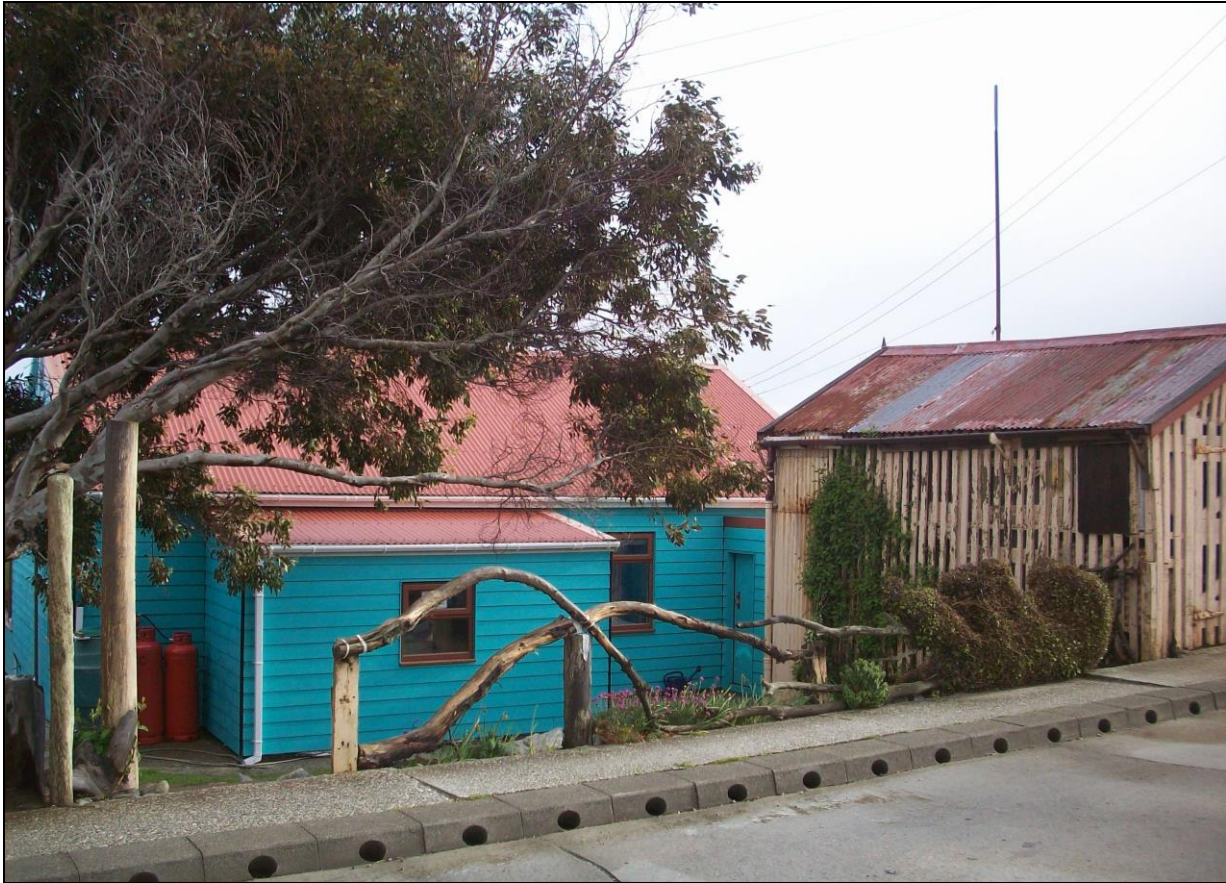
5 St Mary's Walk from the south December 2020 - JCNA
