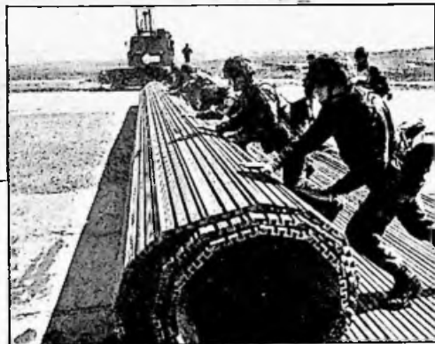
Above - Concrete blocks are used for strategic repairs on runways used by heavy aircraft such as TriStars. Right - Matting, on the other hand, is rolled over a dummy crater filled with hardcore in a tactical repair for emergency work on runways used by lighter aircraft
