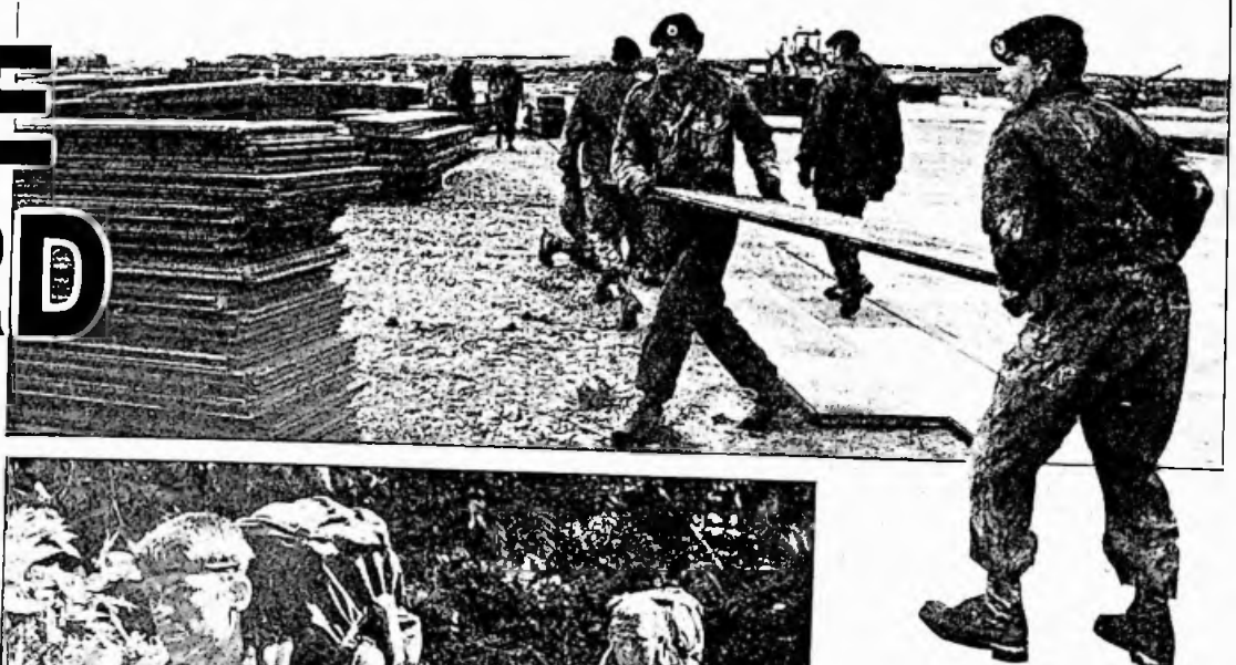
Sappers from 35 Engr Regt tear up the fabricated runway surface constructed at RAF Stanley
