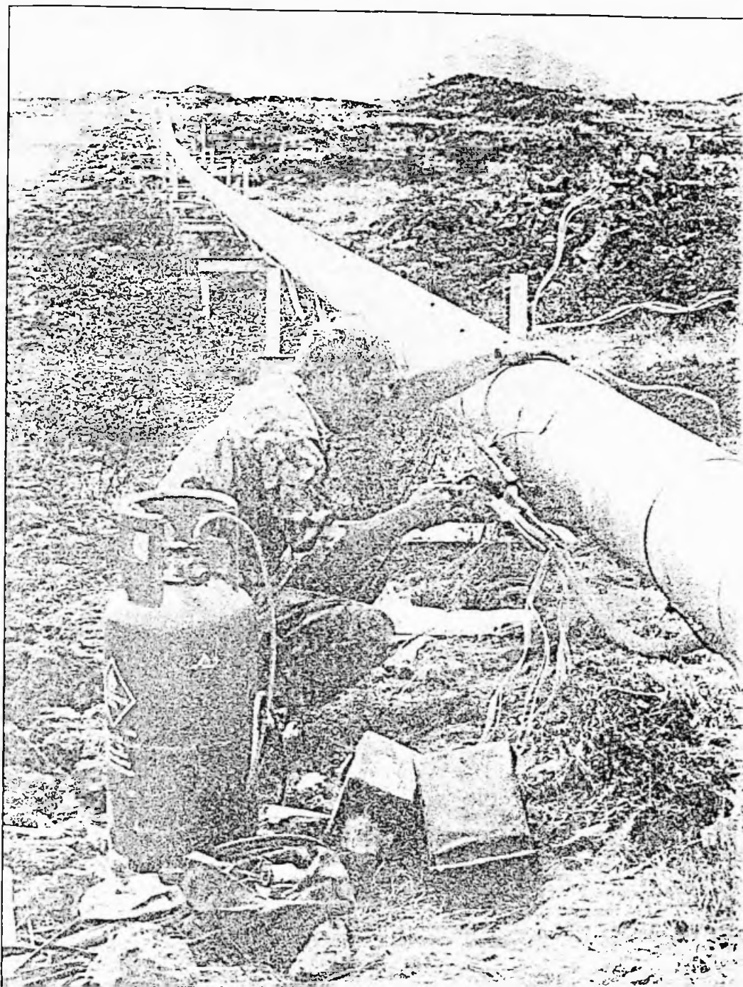
Heat-shrinking a waterproof cable joint hanging beneath the main aviation fuel pipe to the airfields on Ascension Island
