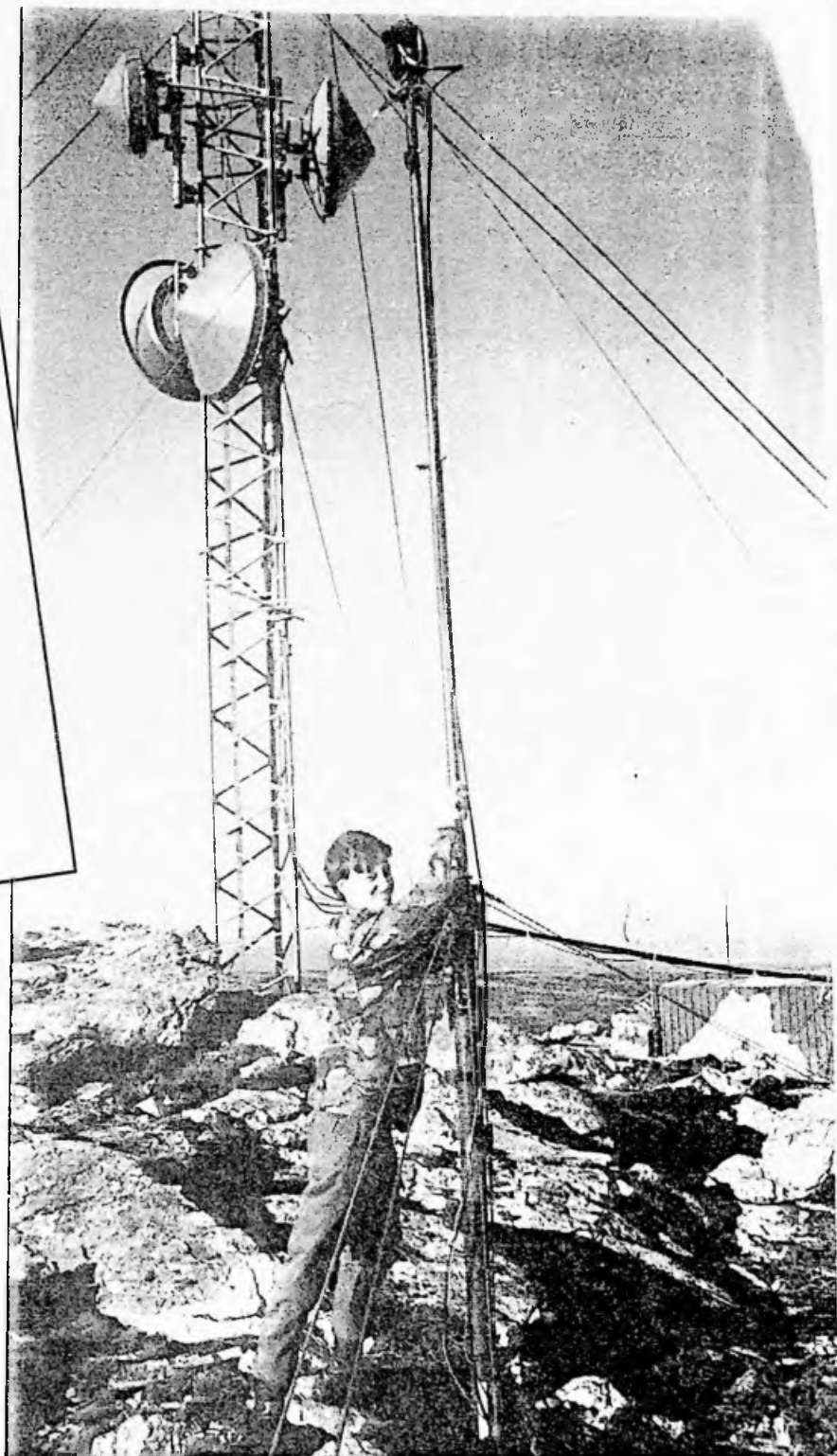
On hill tops where the wind can reach hurricane force, the slightest error in mast siting, or a loose guy rope, can mean a loss of communications. Sig Dave Cooke makes good use of a sunny spell to begin some routine maintenance
