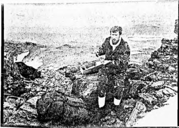
Ship's Met. officer Lieut. Chris Pardoe checks and resets a high-low thermometer which has been kept in place on an Antarctic peak for 70 years. Highest temperature recorded was 76F, lowest minus 10C.
