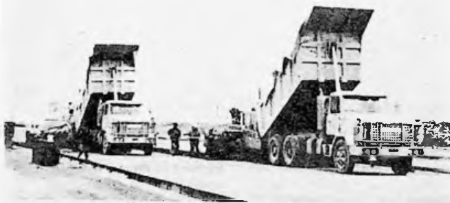
Two Leyland and Landtrains are being used with Blaw Knox pavers on the main runway for the Mount Pleasant airfield in the Falklands
