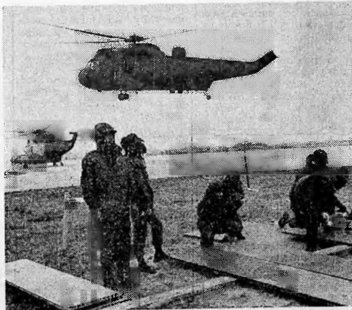
Laying of the matting that is intended to cover all of Port Stanley airfield.
