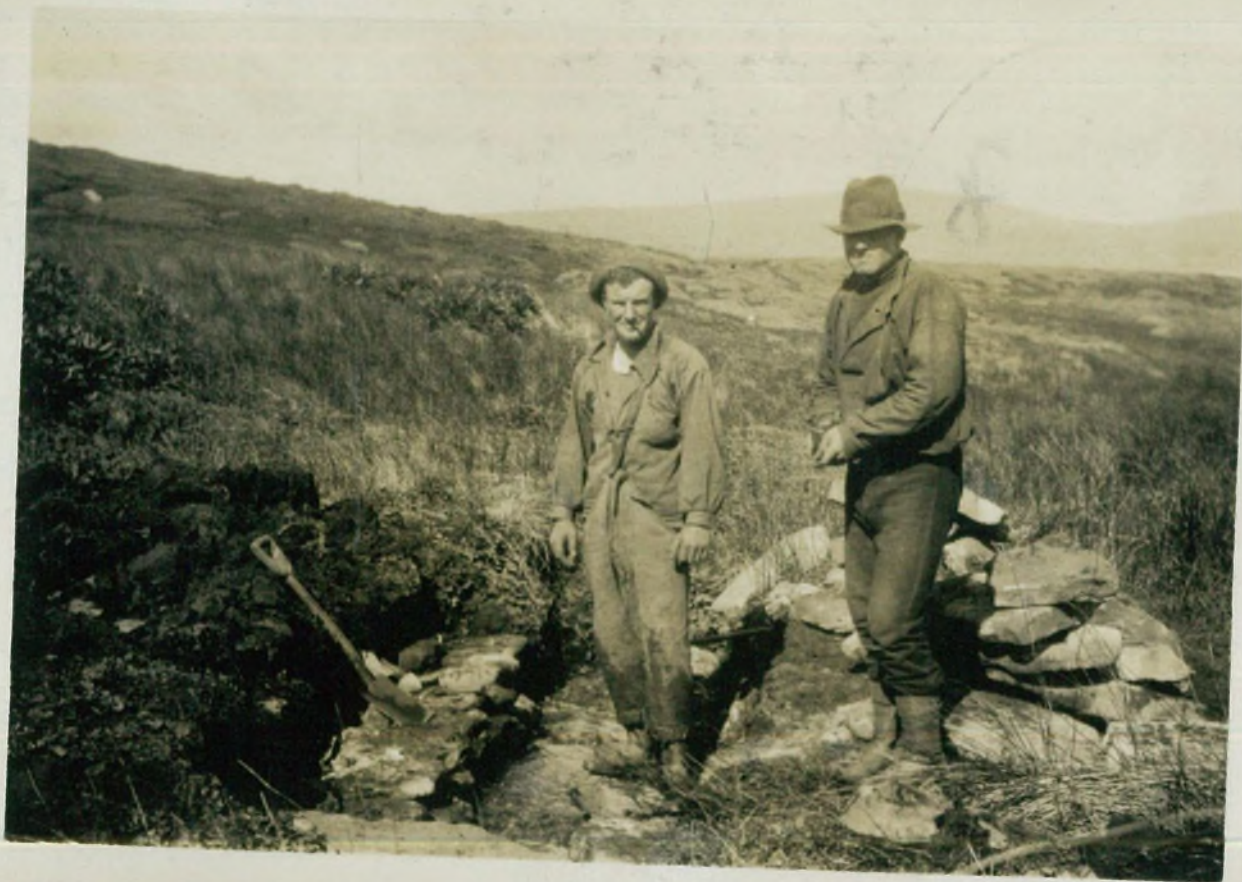
D. Goodwin - building Stone Bridge W. Brown Sep 1930
