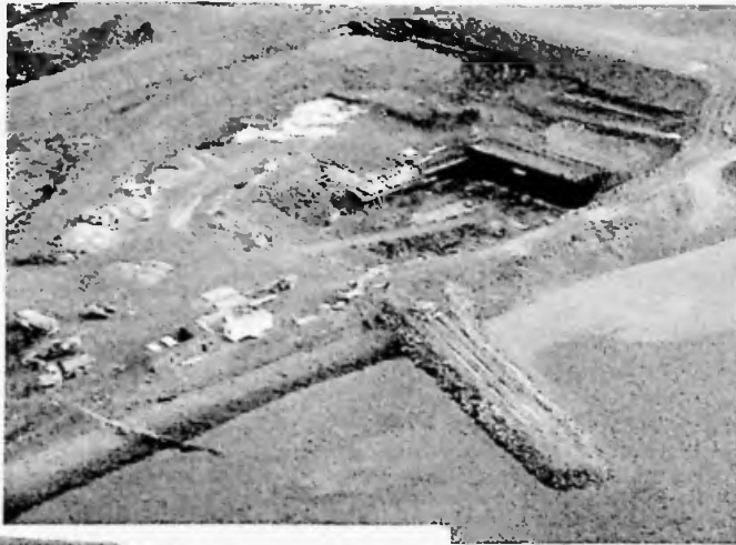
Above: New Haven ferry head takes shape with the shallow water area left to dig out by the PWD gang, visible to the right of the breakwater; Left: The Morrison (Falklands), constructed concrete ramp nears completion. The bottom of the hole is approximately five metres below sea level.
