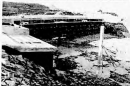
Above: New Haven ferry head takes shape with the shallow water area left to dig out by the PWD gang, visible to the right of the breakwater; Left: The Morrison (Falklands), constructed concrete ramp nears completion. The bottom of the hole is approximately five metres below sea level.
