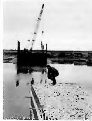
Above: Work gets underway on Boxer Bridge.
