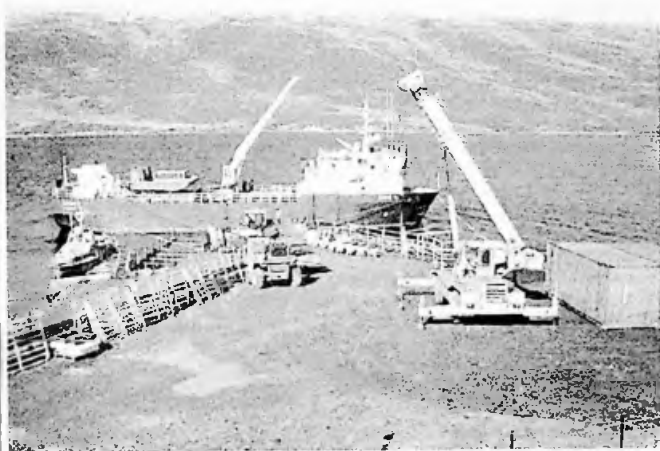
Above: Tamar FI at Port Howard this week as work gets underway at the jetty to build a ramp for ferry operations. Picture: R Macaskill
