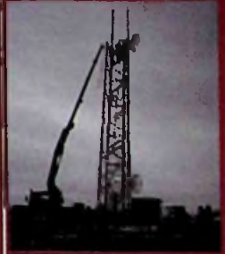
Building Goose Green Tower
