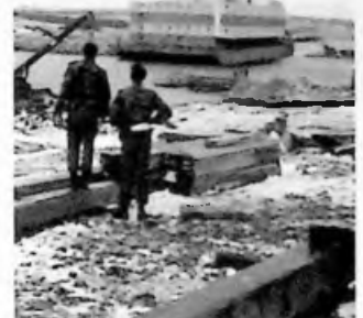
Above: One of the coasteal accommodation units is manoeuvred into place at the Canache.
