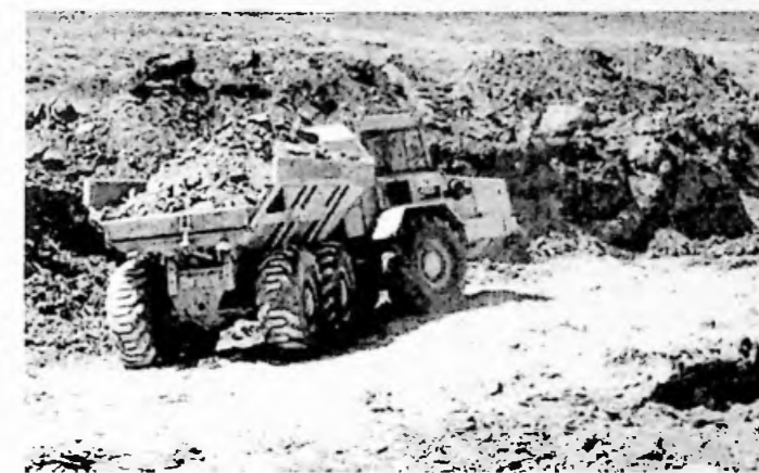
Above: North Camp Road construction
