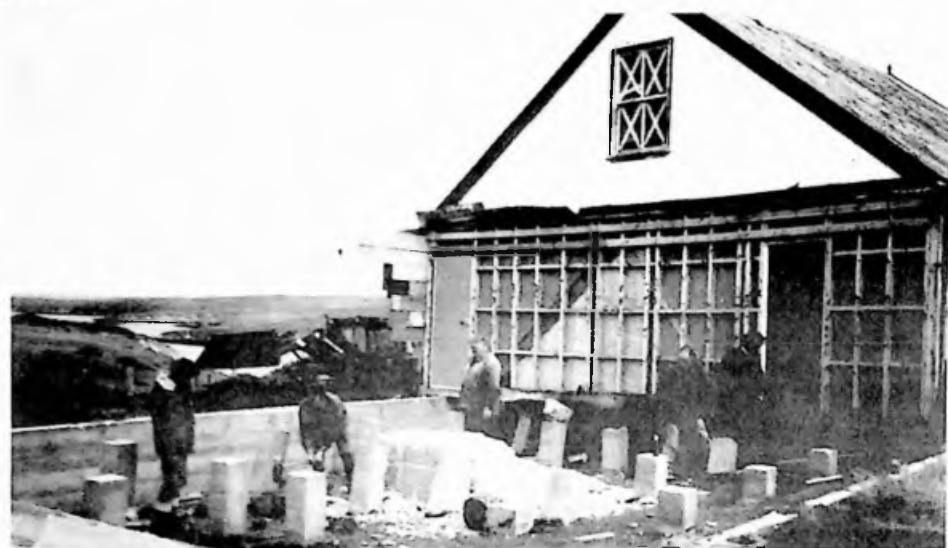
STAGE ONE: Moving the house off its original foundations at Roy Cove
