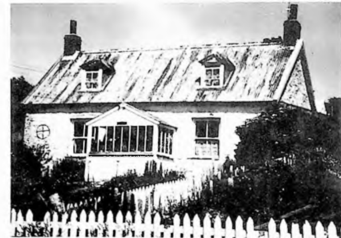
A well proportioned traditional stone cottage at 21 Fitzroy Road which illustrates the suitability of simple symmetrical sash windows. The brick chimneys which have been retained add balance to the building.
