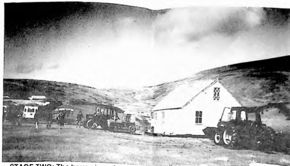
STAGE TWO: The house is on its sledge and the towing tractors are ready for the off
