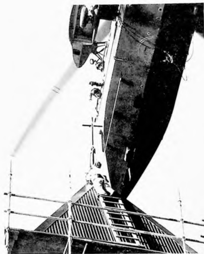
ABOVE: While the pilots hold the Sea King breathtakingly close to the spire, the helicopter winchmen carefully lower the cross down
