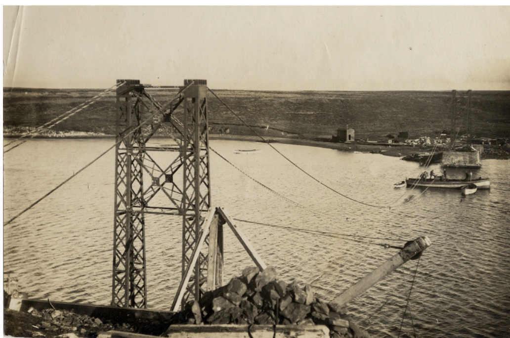
LEFT: FC-004-0053. BODIE BRIDGE. PUTTING SUSPENSION WIRES OVER CREEK.
