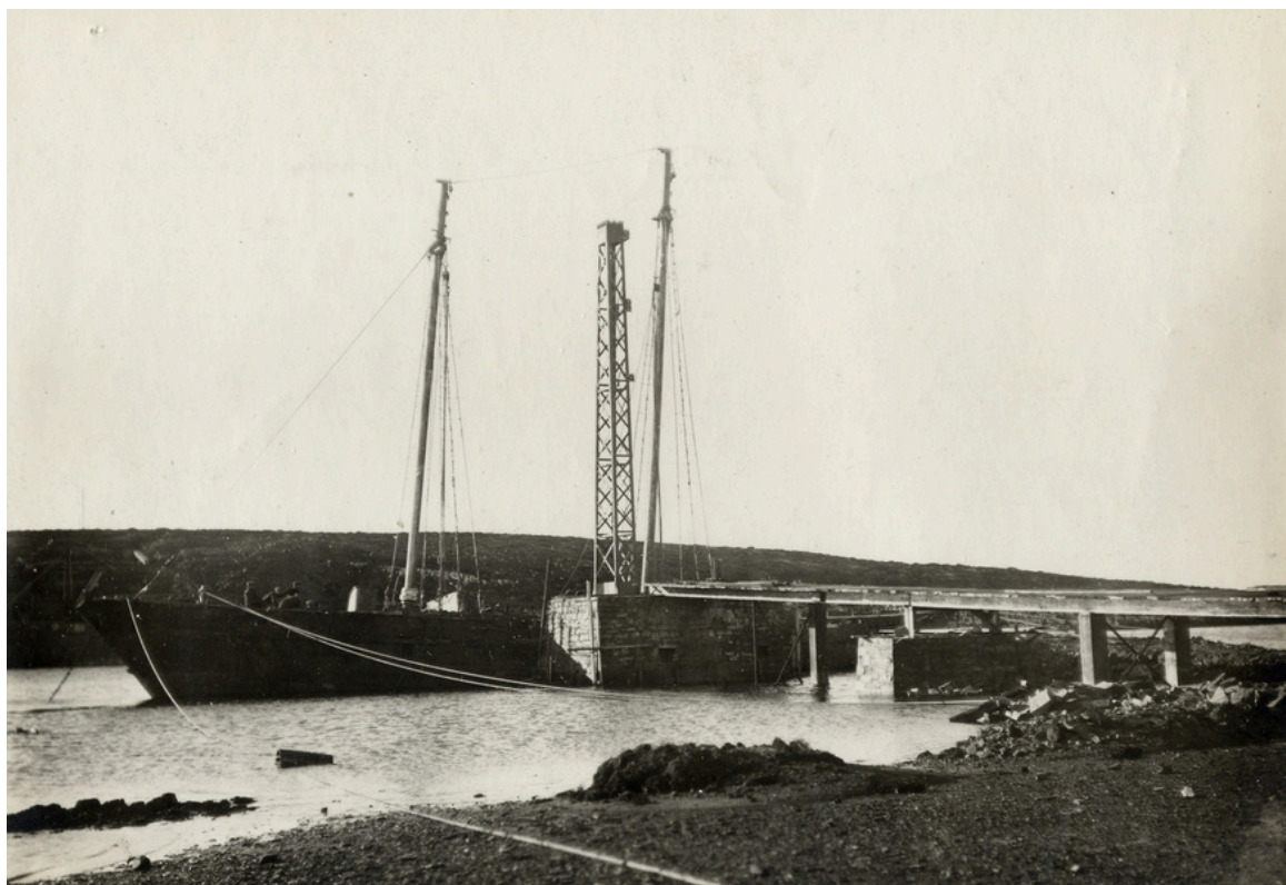
ABOVE: FC-004-0048. BODIE BRIDGE. FINDLEY CREEK ABUTMENT WITH 'LAFONIA' ALONGSIDE AND ONE TOWER ERECTED
