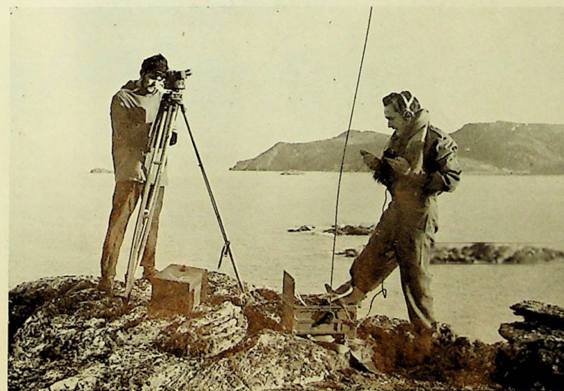
SURVEYORS FIXING POSITION WITH SUN-SIGHT AND TIME SIGNAL, SIGNY ISLAND, SOUTH ORKNEY ISLANDS
