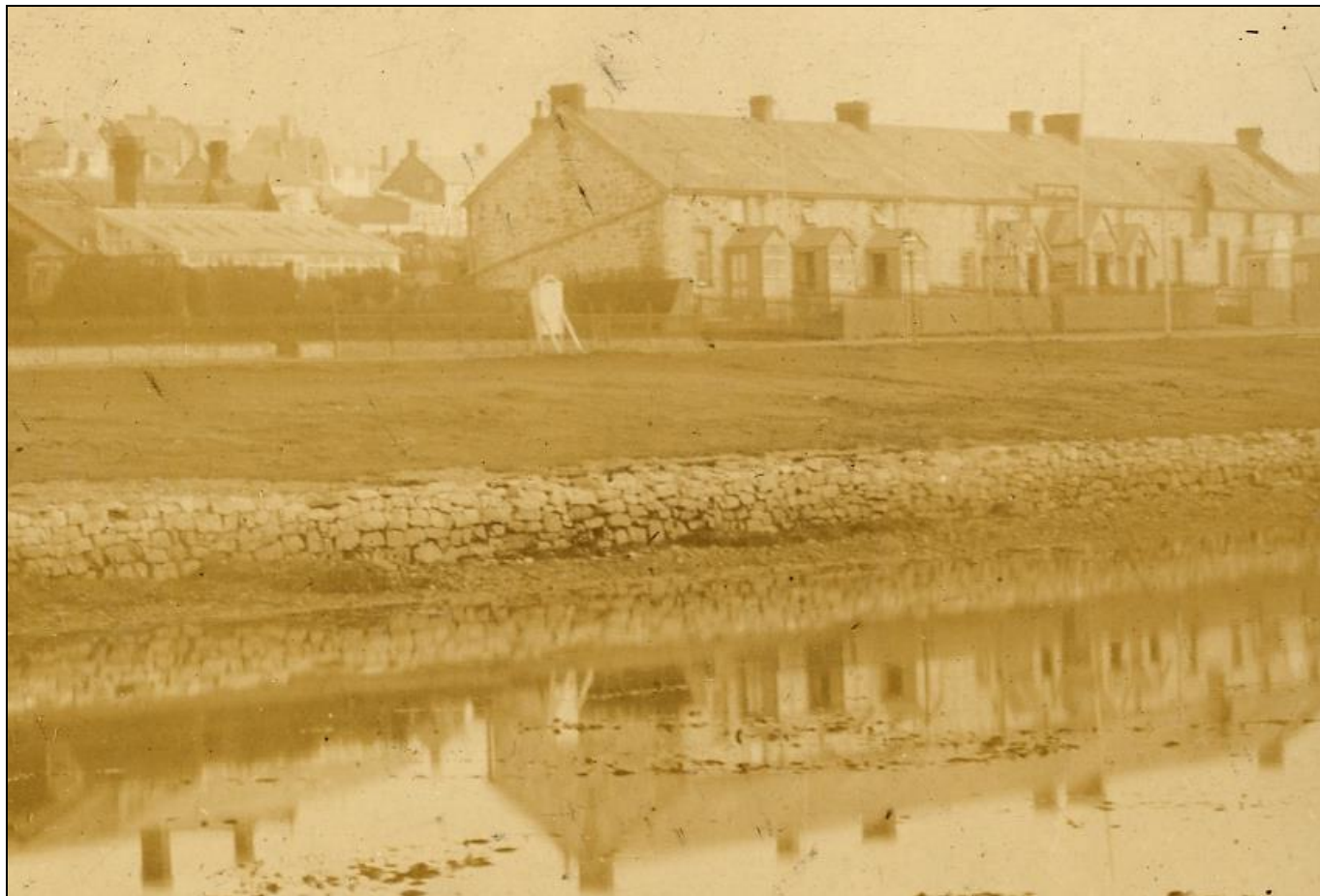
From the North East Circa 1890s – with the addition of porches
