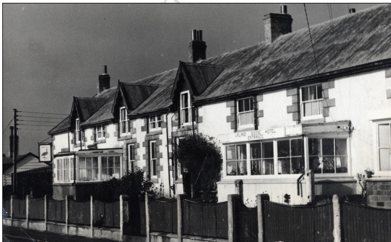
From north west
