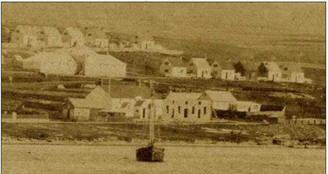
1863 – Second house from the right middle row
