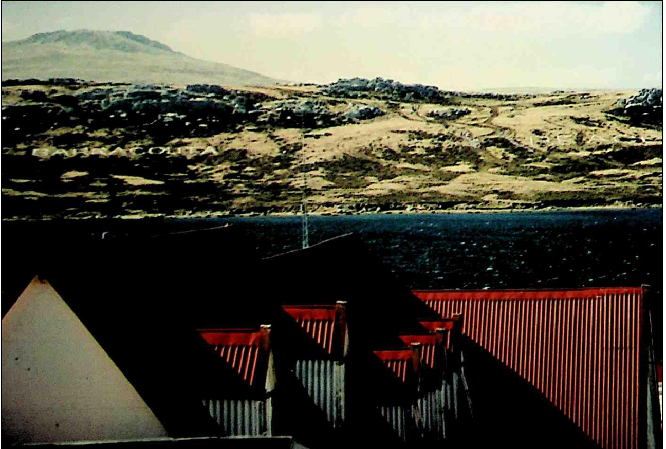
1993 - From the south showing the different roof lines and dormers
