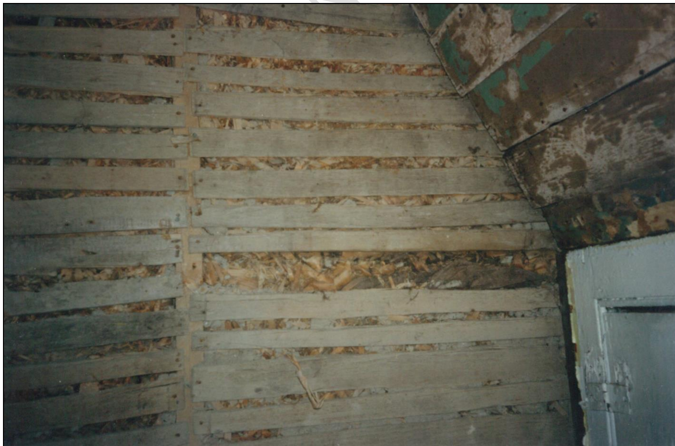
Lining and insulation, photographs circa 1990 - JCNA
