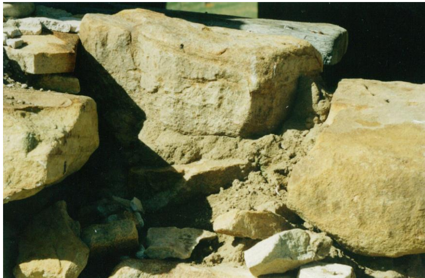
Undressed stone with clay mortar in Barnard's House
