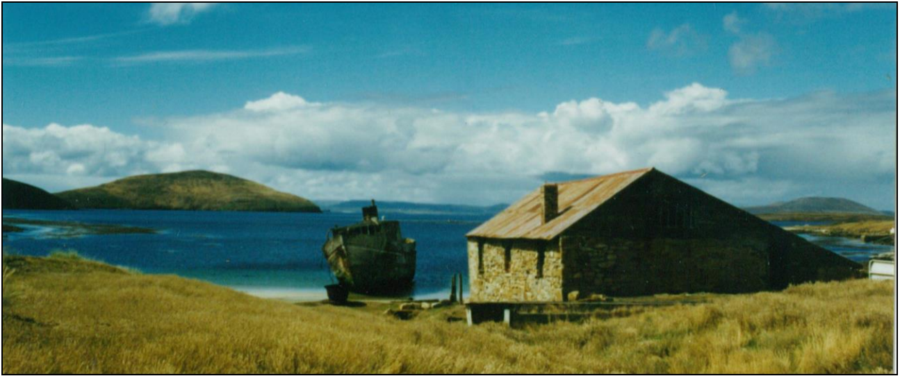
Barnard's House in the 1990s – different uses over the years have resulted in additions and modifications
