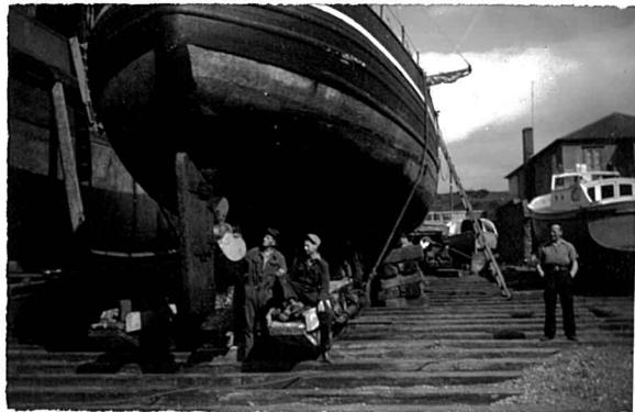
Slipped at Renter Area now
