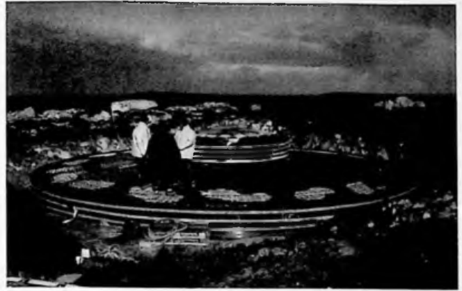
Above: One of the concrete tower bases at the Sand Bay wind farm (Picture: T Heathman); Below: The modest looking Waste Heat Recovery plant, which will save thousands of litres of fuel a year.
