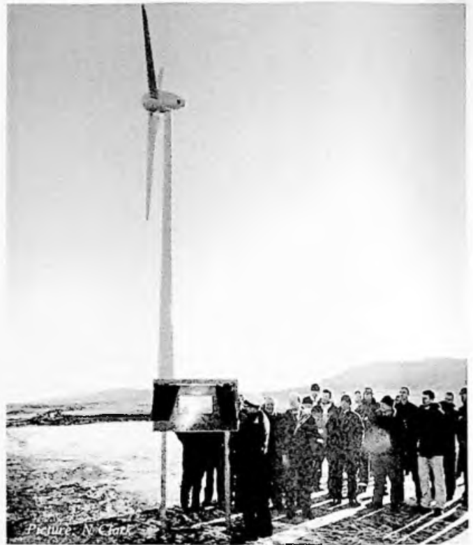
One of three majestic wind turbines under construction.
