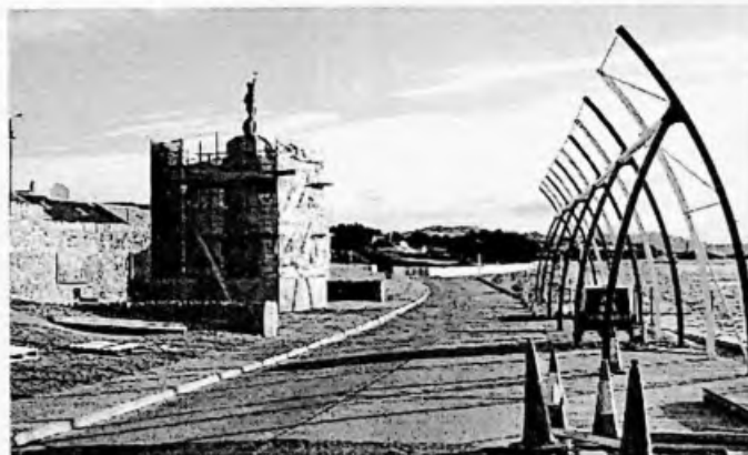
Above: The shelter still under construction, opposite the Liberation Monument, which is being renovated.
