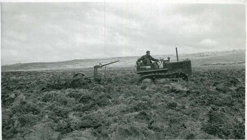
Cross ploughing on "60 acre" with three furrow disc plough and Department tractor. Photographed autumn 1944.
